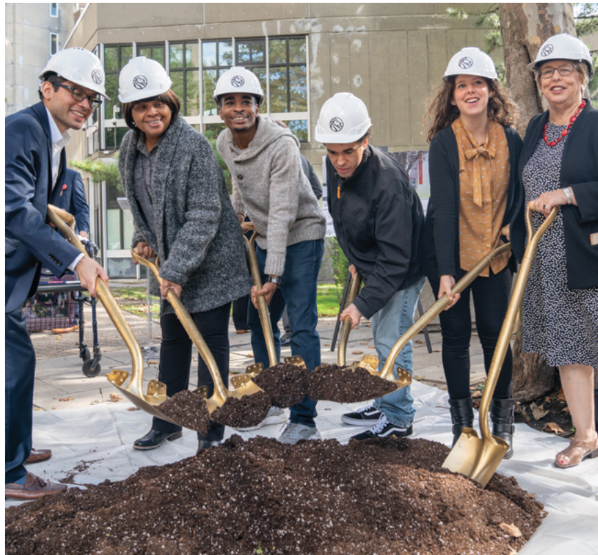
In October 2018, the Library broke ground on Roosevelt Island for a new library building. The updated Roosevelt Island branch will have more community space, a children's room, and technology upgrades.
